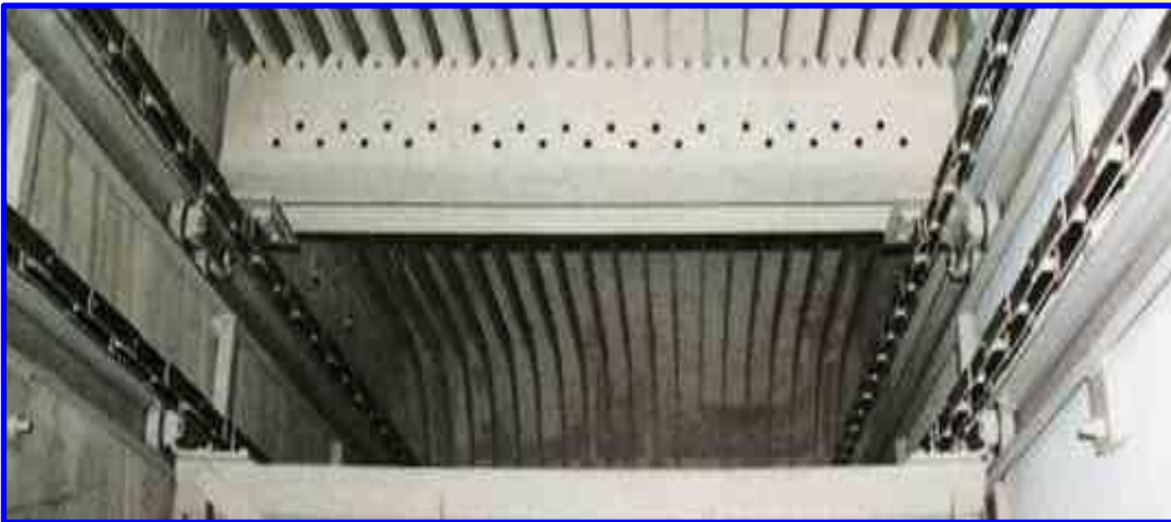
MACH Bar screen Installed at Miami-Dade WWTP, FL
